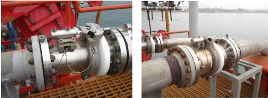
*Shown is a Dual release ERC incorporating both a Cable and Hydraulic Release.*
